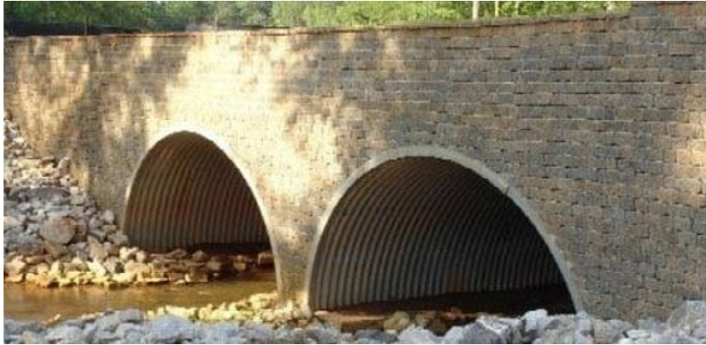
Figure 21 Example of a Culvert Bridge
