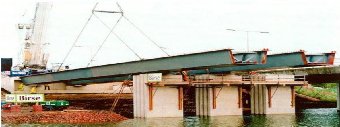
Figure 30 Open Trapezoidal Composite Box Girder during Construction
