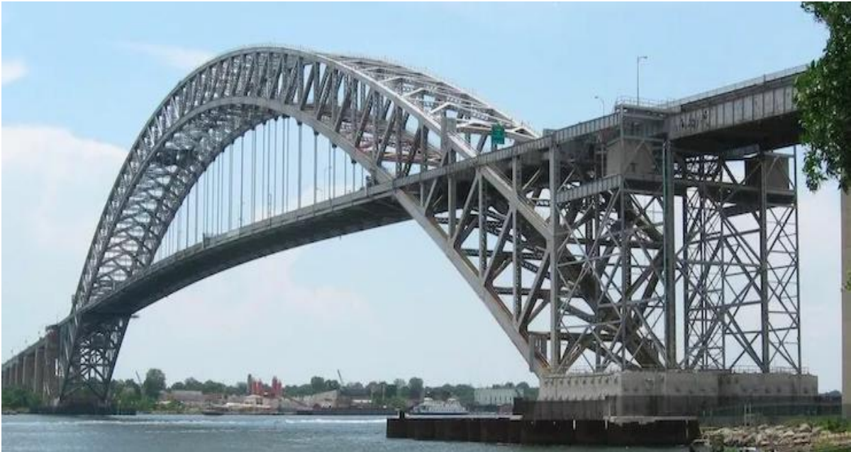
Figure 26 World's 5 th Longest Steel Arch Bridge | Bayonne Bridge
