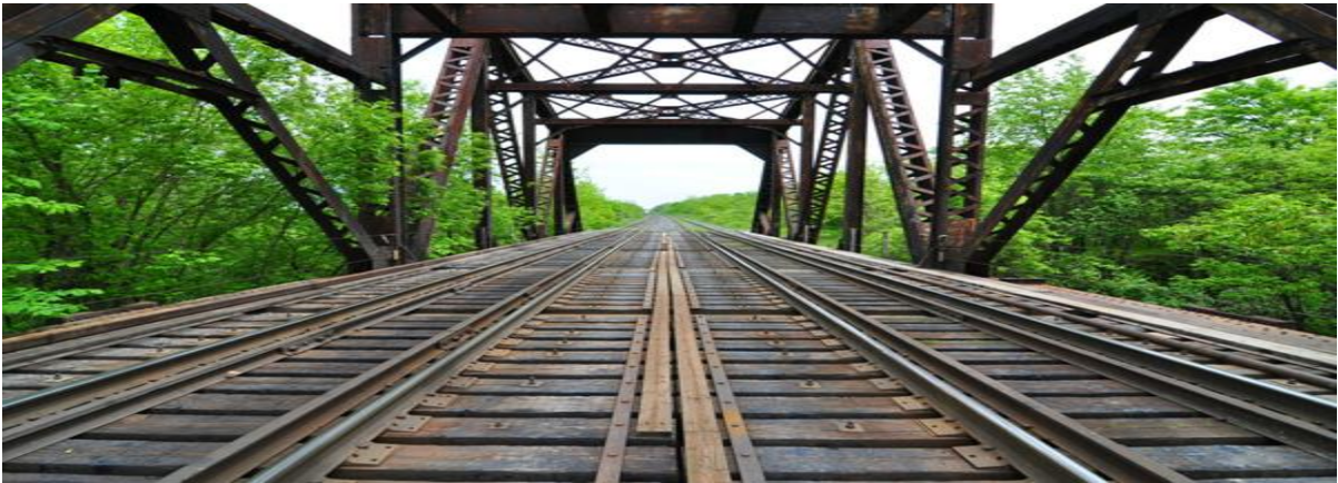
Figure 18 Example of a Train Bridge
