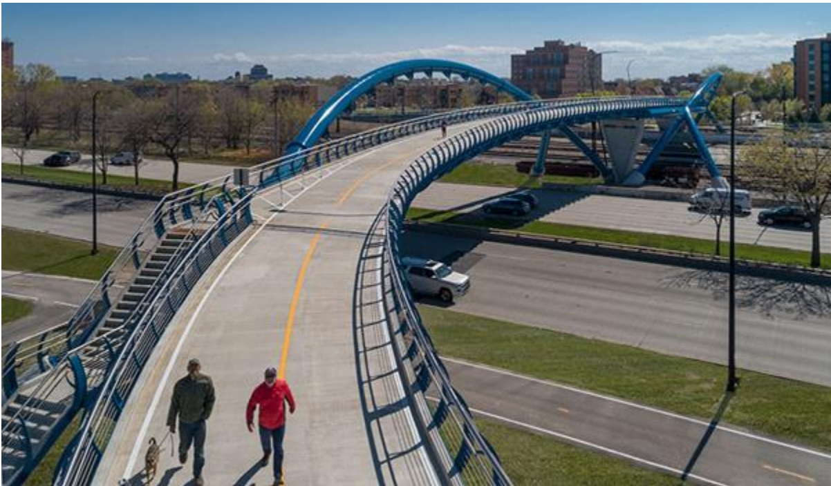
Figure 16 Example of a Pedestrian Bridge
